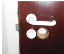
Left: the main bar had no smoke alarm; above: smoke alarms were missing throughout the hotel and fire doors had holes in them
